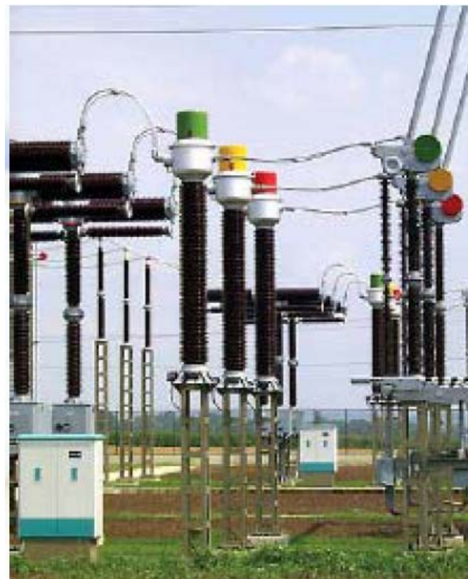
(b) Current transformer (CT)
